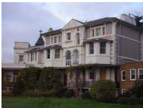
Figure 1 Western Elevation of Building A
