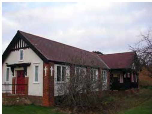
Figure 17 Building I Showing Eastern Entrance Porch
