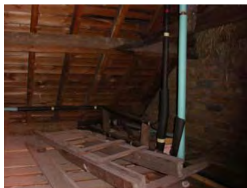
Figure 18 Roof Void of Building I
