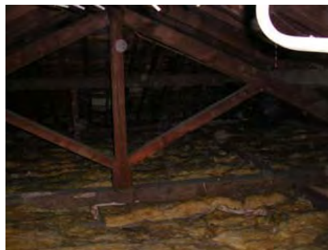
Figure 4 Roof Void in Building A
